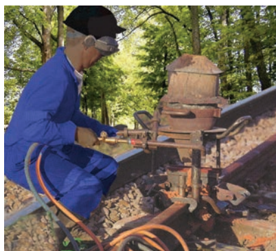
Figure 3.11 Thermit process for joining railway tracks
